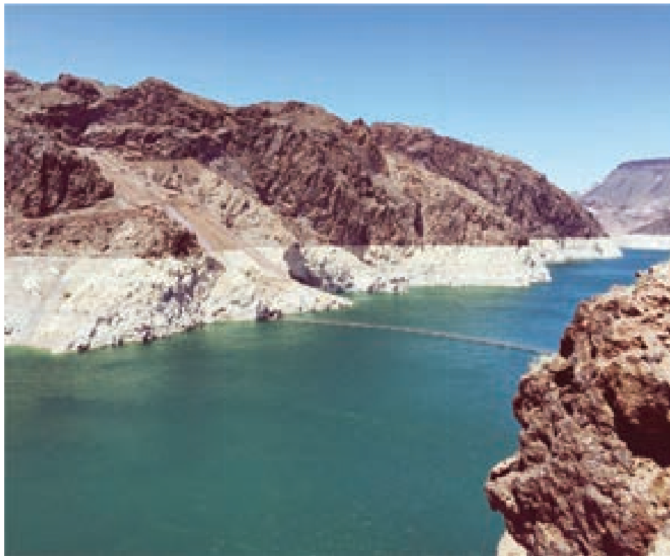
The Hoover Dam, Nevada, USA Light-colored rock indicates previous water levels within the dam due to drought. Source: Arlen Stawasz
