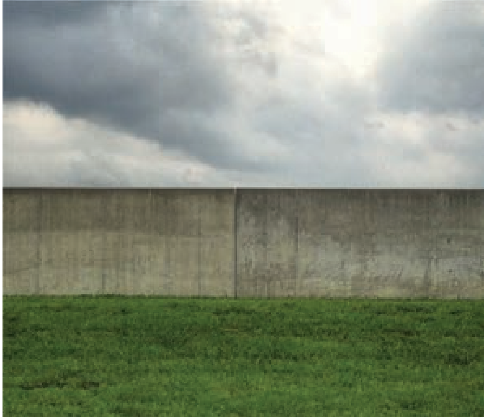
Portion of the levee prior to Katrina, about 20 feet high. Source: Arlen Stawasz
