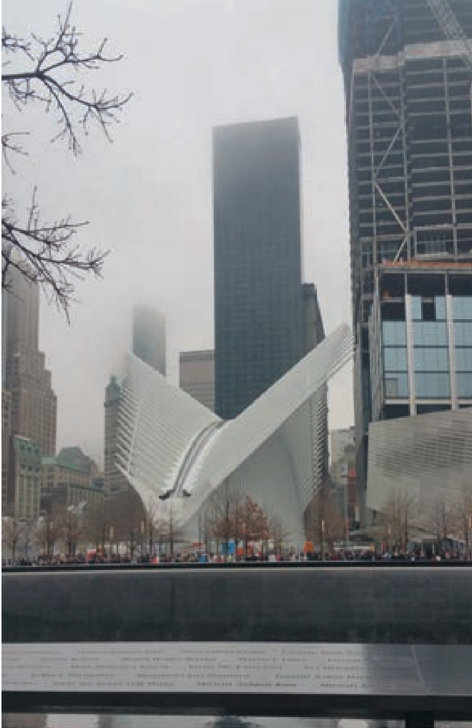
View of newly constructed World Trade Center transit station designed by Santiago Calatrava. Source: Eric Kaufman (2016)
