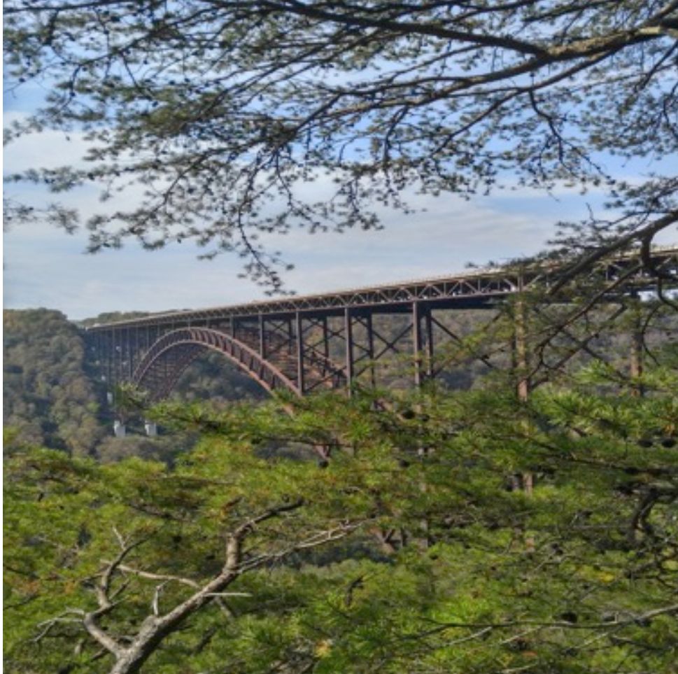
New River Gorge Bridge completed in 1977. Source: Eric Kaufman (October 2016)
